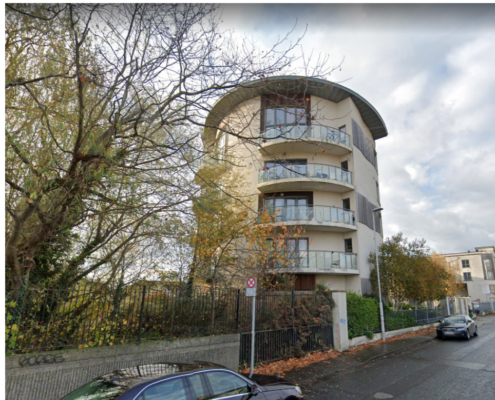
8 - View From Richmond Road of Richmond Hall Apartments
