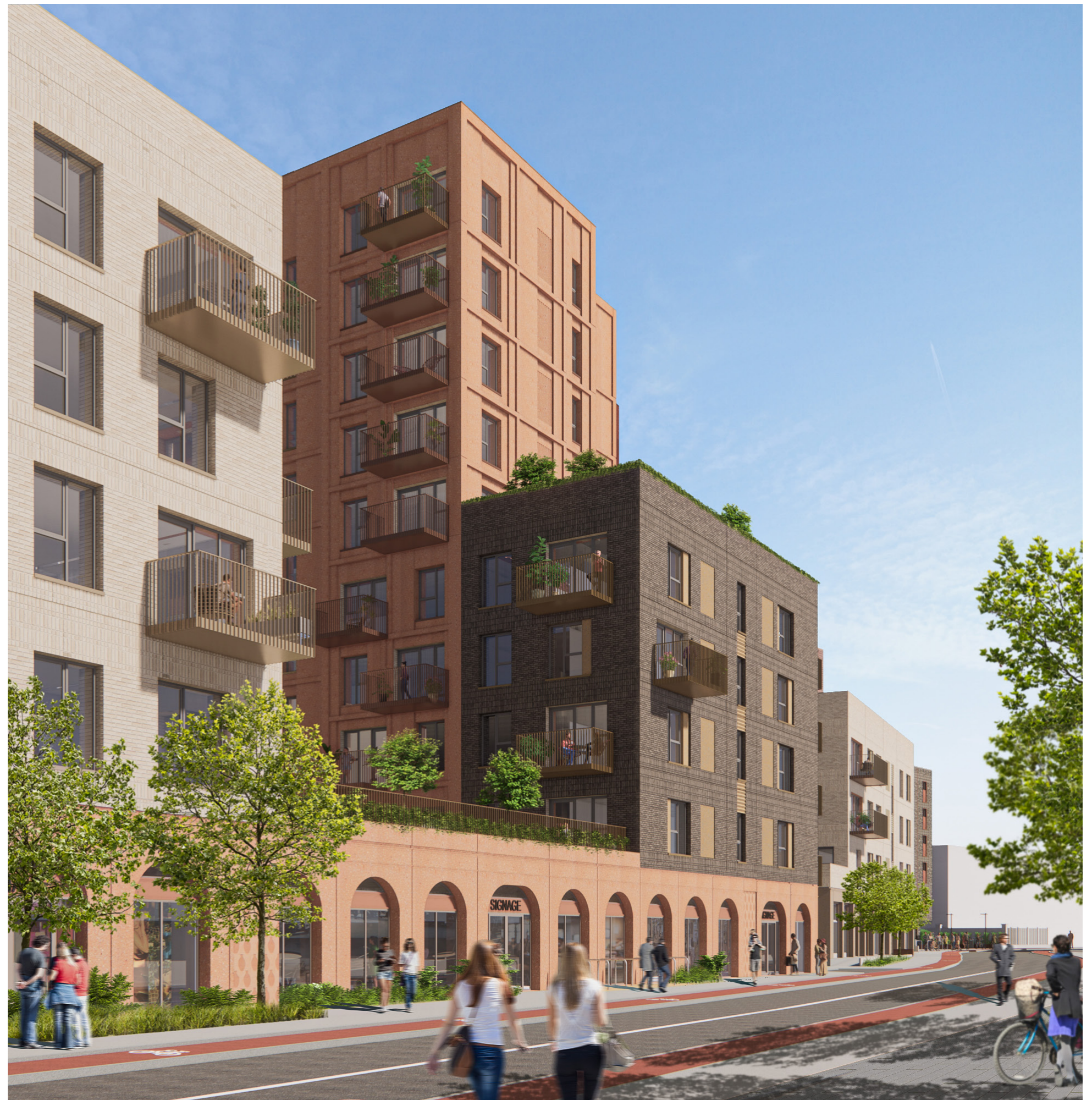
View Down Richmond Road
