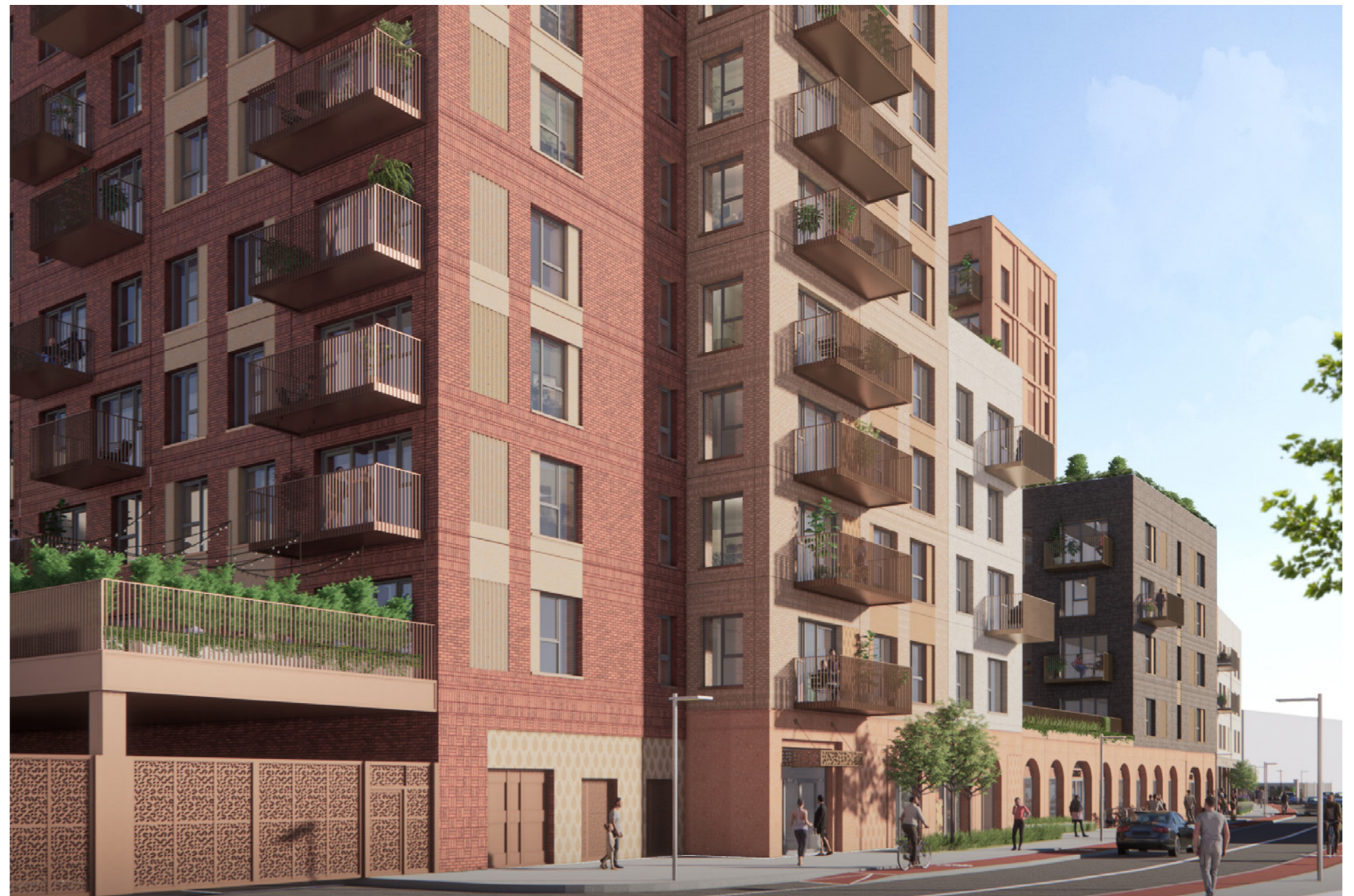
View Down Richmond Road
